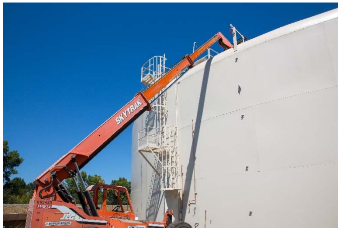
Detail Work on Trimble Reservoir
