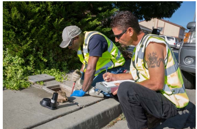
Meter Replacement Project
