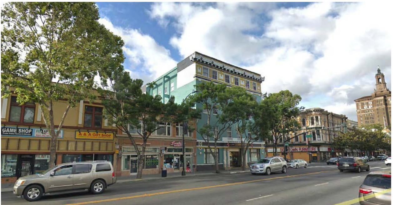
Picture 3 View of E. Santa Clara Street looking west toward the Bank of Italy building and the edge of the Historic District. The five-story building in the center is the former YMCA, now Hotel Clariana.
