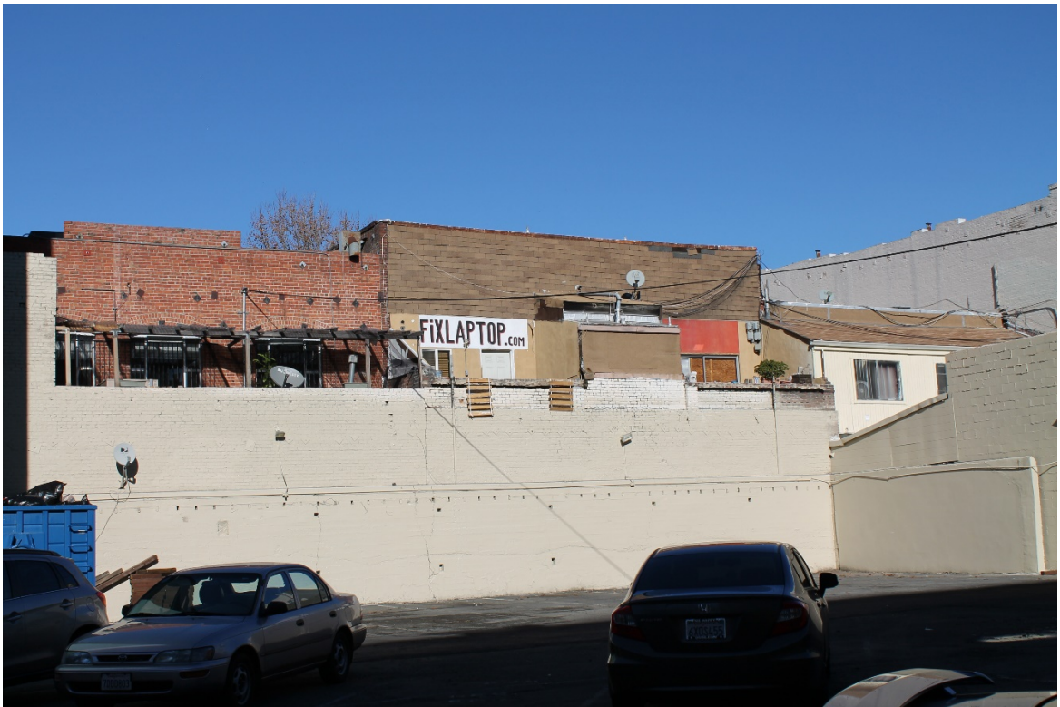
Picture 6 View of the rear facades of the historic buildings between S. Fourth St. and S. Third St. on E. Santa Clara St.
