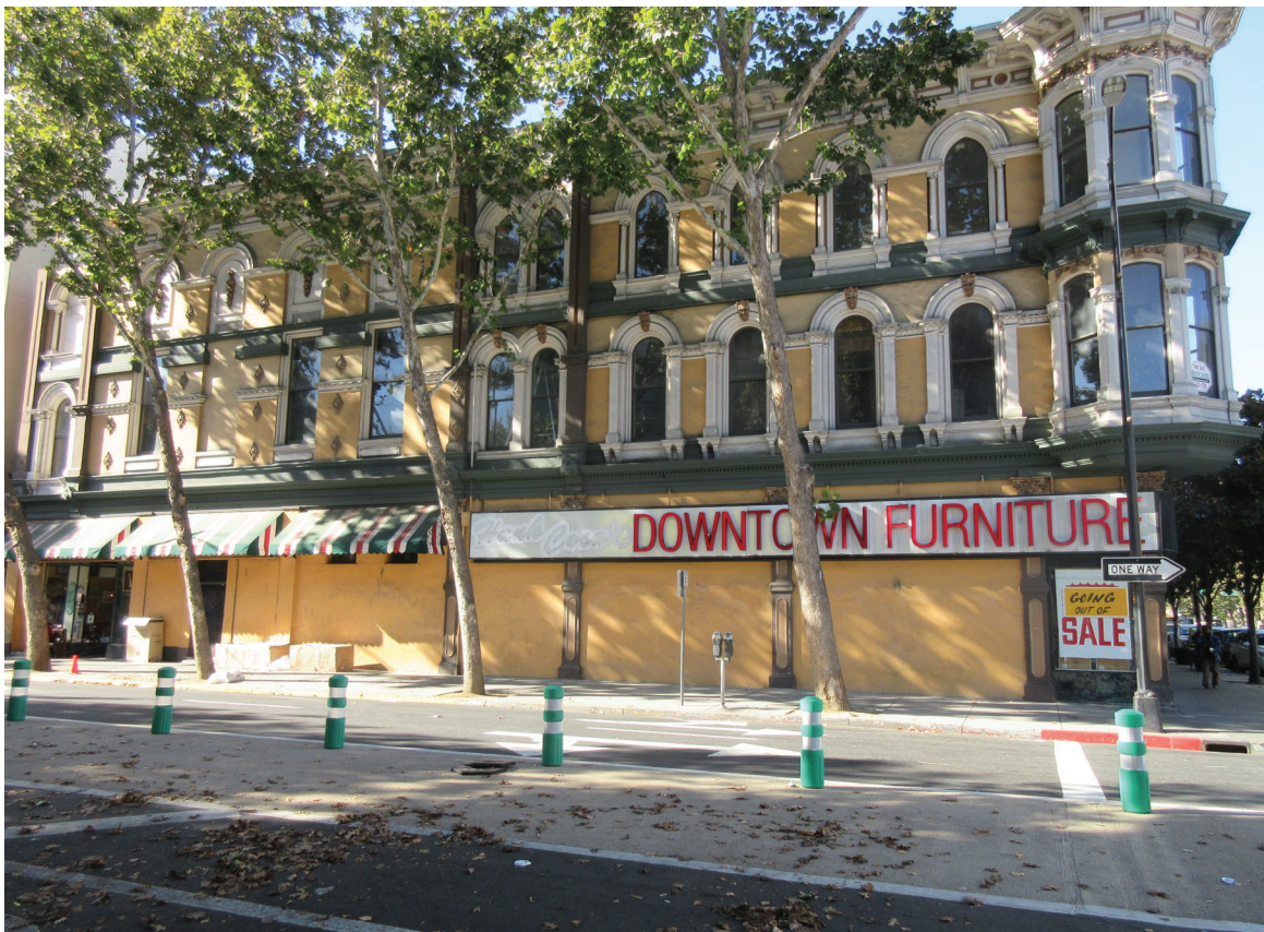
Photo 6 - View of surrounding development, looking west on South Third Street.
