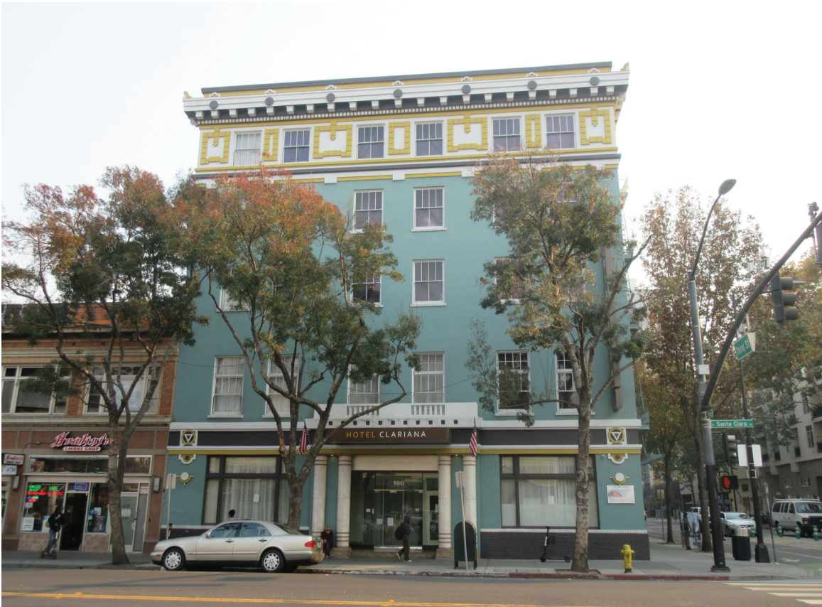
Photo 1 - View of project site, looking south on East Santa Clara Street.
