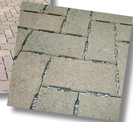
**Bottom right: Permeable interlocking concrete pavement is arranged in a grid pattern. Joints are filled with aggregate to allow infiltration between the pavers.**
