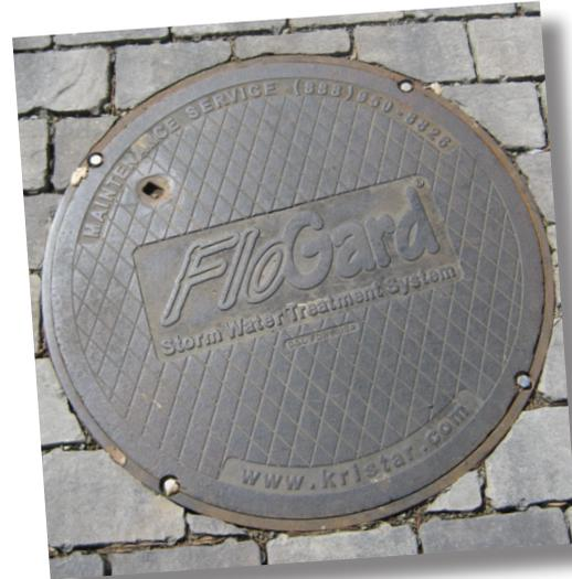
**Above: Mechanical Stormwater Treatment Measure, Manhole Cover**
