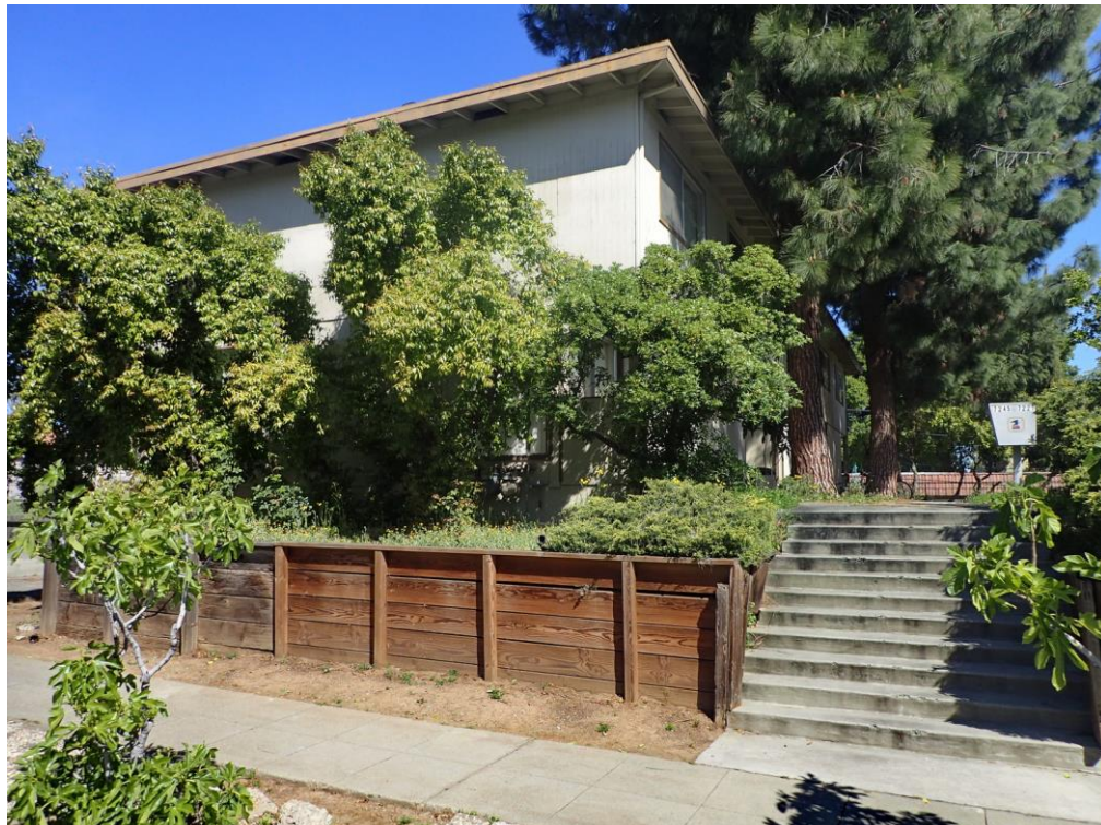
Front of 7245 Bark Lane at site entry, viewed facing north.
