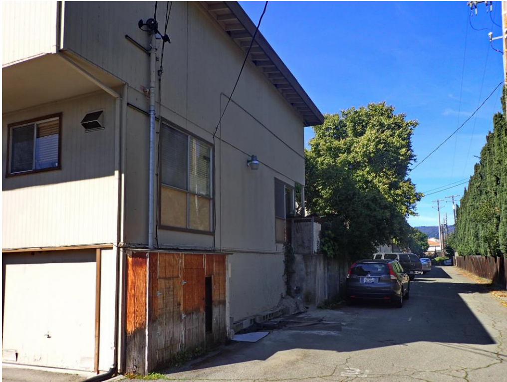
Rear of 7201 Bark Lane at rear driveway, viewed facing west.
