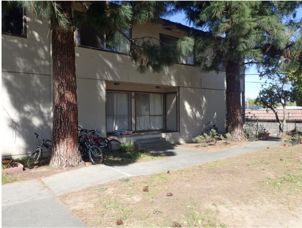
7245 Bark Lane, typical entry alcove, viewed facing northwest.
