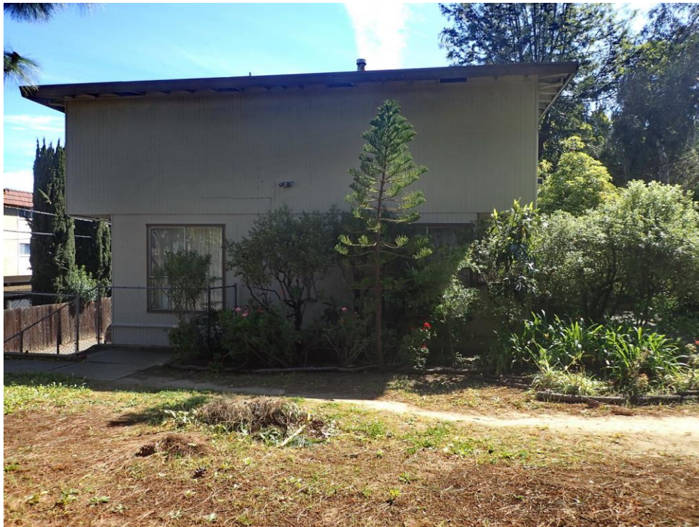
Side elevation of 7221 Bark Lane, viewed facing east.
