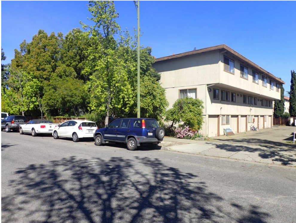
7201 Bark Lane overview, viewed facing northwest.
