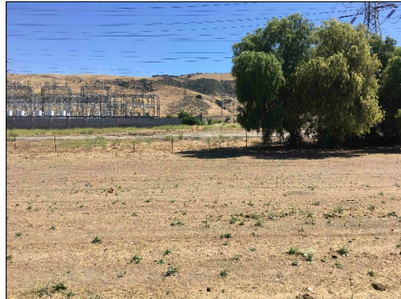
Photo 4. Disturbed annual grassland in between the riser pole and the Metcalf Substation where trenching for the transmission line will occur.
