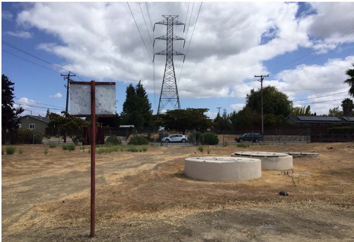
Site Challenges: PG&E aerial utilities and SCVWD pipeline infrastructure.
