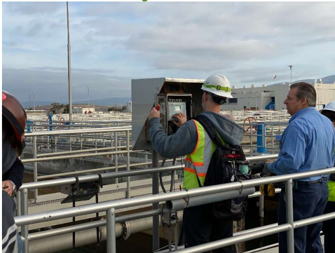
Figure 4: The contractor performs electrical instrumentation adjustments and verifies readings with an existing distributed control system (DCS) node.
