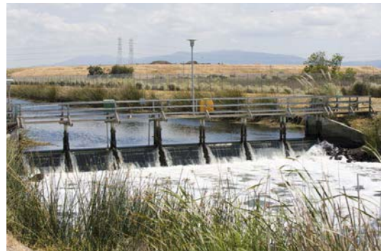
Treated Water Flows to the Bay
