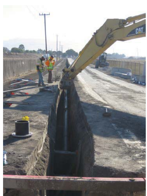
Force Main Installation
