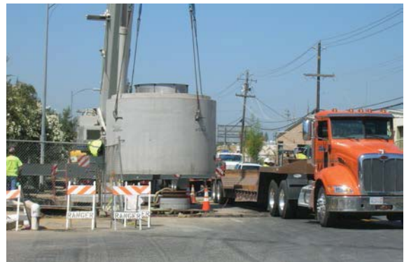
Installation of Large Trash Capture Device on 7 th Street
