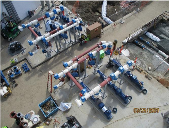
Figure 9: The upgraded foam suppression and withdrawal pumps and visible piping for thermophilic Digesters 5 and 7.
