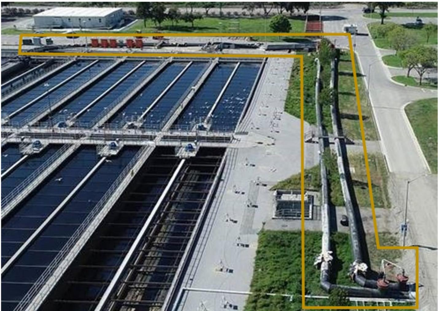
Figure 5: 78-Inch SES Reroute System Outlined in Orange
