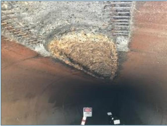
Figure 3: Rebar degradation of 96-inch SES pipeline
