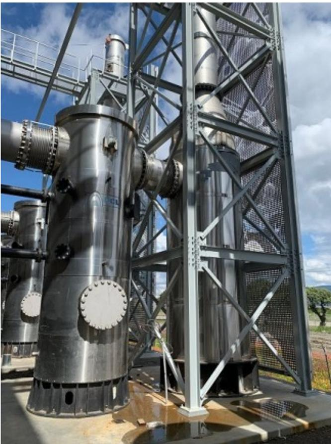
Figure 8: The new engine generators' high exhaust heat is used to produce hot water, which is then used to provide heat to the digesters and other facilities. The exhaust gas is cleaned through a treatment system before being discharged through the exhaust stacks.
