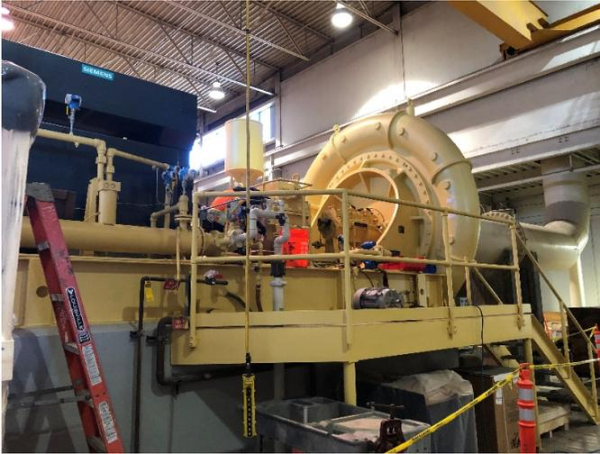
Figure 2: Reoriented and refurbished mechanical system, including a new motor and various utilities connections, for one of the blowers in the Power and Air Building.
