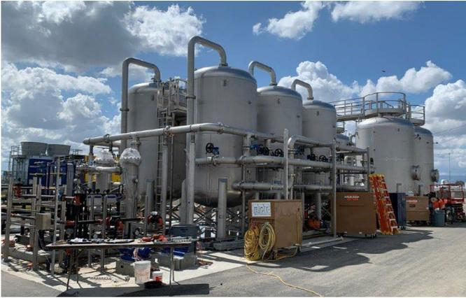
Figure 6: New gas treatment system which cleans impurities from the digester gas prior to being used by the internal combustion engines to produce electricity and heat.
