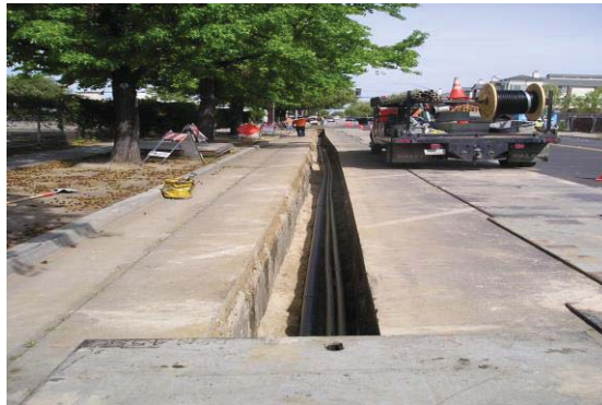
Installation of Utility Conduits (Japantown)
