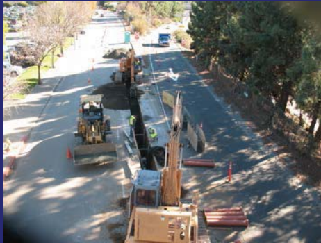
Parkmoor Sanitary Sewer Replacement Project
