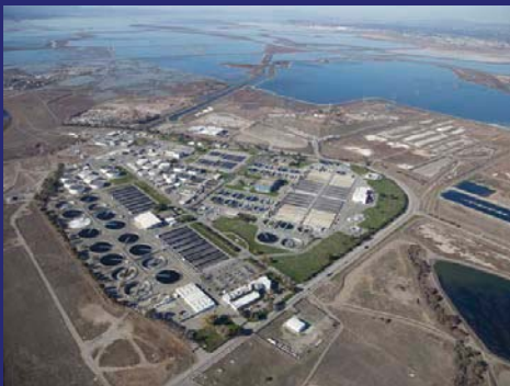
Water Pollution Control Plant
