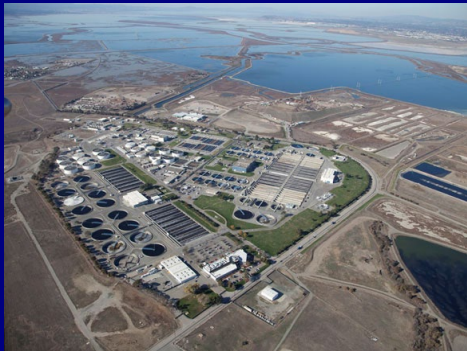
Water Pollution Control Plant
