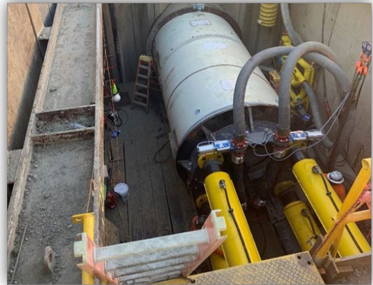
Fourth Street 84-inch Interceptor Phase VI-A
