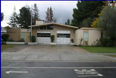
Major Repairs at Fire Stations 4, 14 and 30
