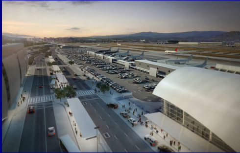
Interim Terminal Facility
