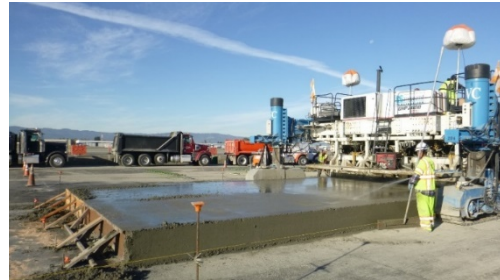
Terminal B Ramp Rehabilitation
