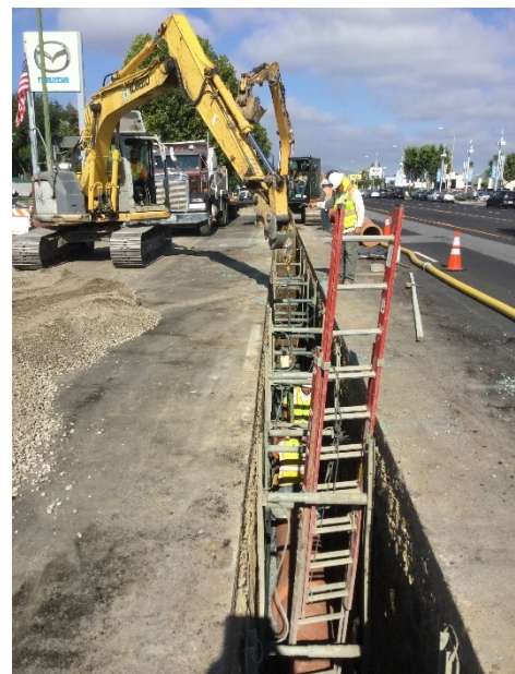
Stevens Creek Sanitary Sewer Replacement
