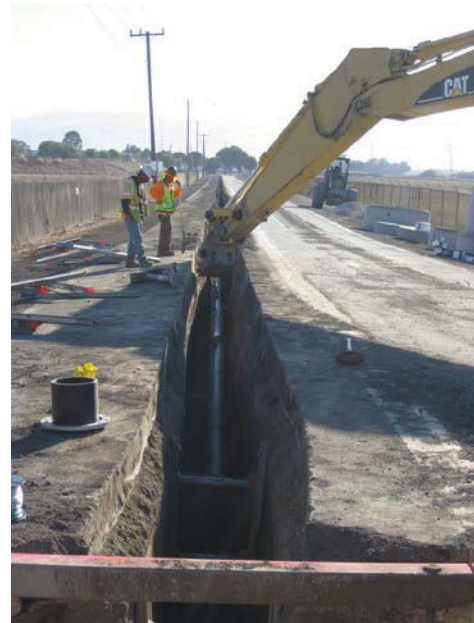
Force Main Installation
