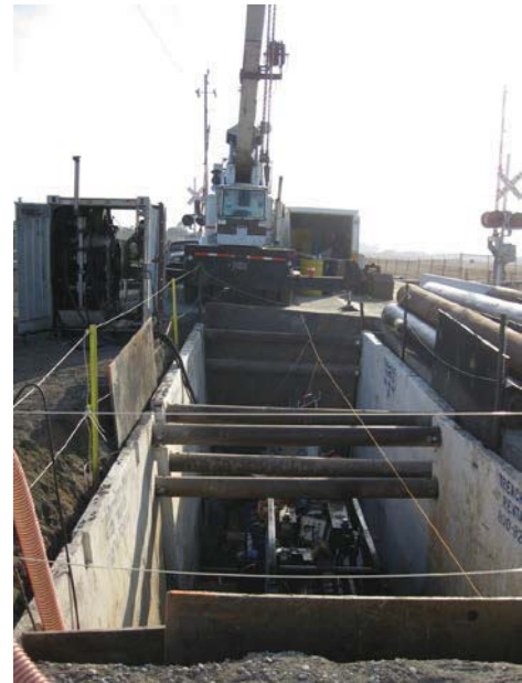
Sewer Rehabilitation by Bore and Jack Operation
