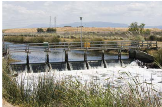
Treated Water Flows to the Bay
