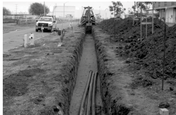
Fire Main Replacement - Phase 2
