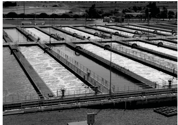
Secondary Aeration Tanks
