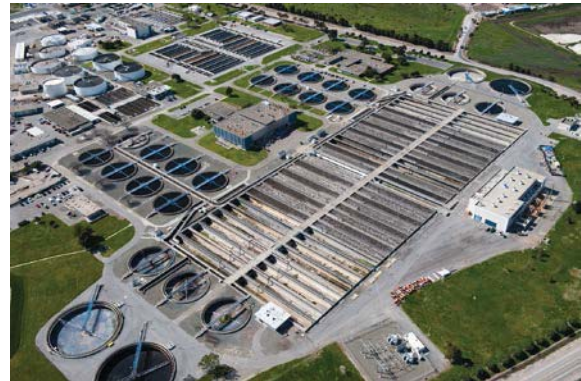
San José-Santa Clara Regional Wastewater Facility
