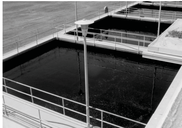
Existing Filter Complex
