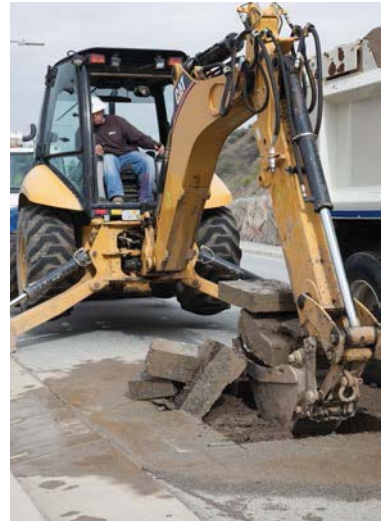
Dove Road Main Extension, Completed in 2013-2014
