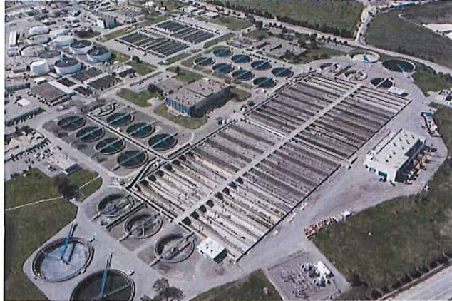
San José-Santa Clara Regional Wastewater Facility
