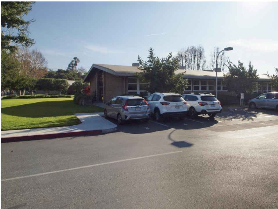
North wing of main classroom building at site entry, viewed facing south.
