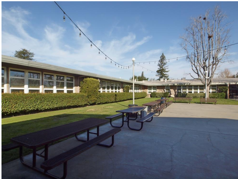
Classroom building from courtyard, viewed facing east.
