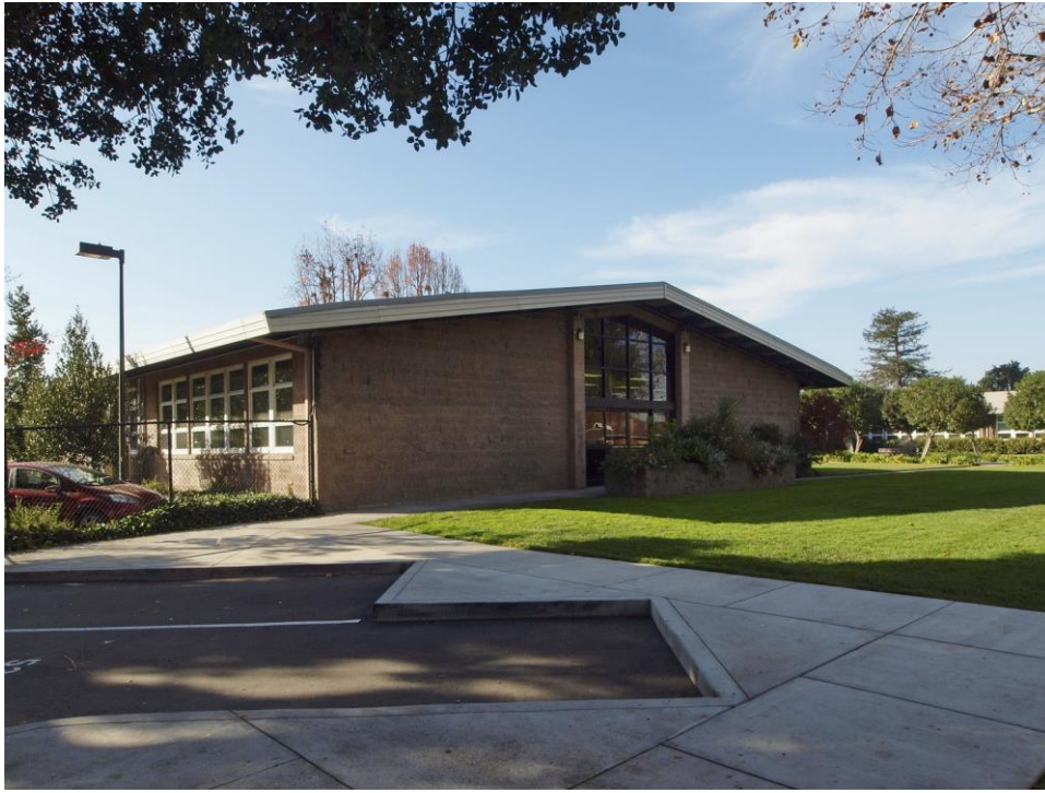
Front façade at Plummer Avenue (south wing), viewed facing northwest.
