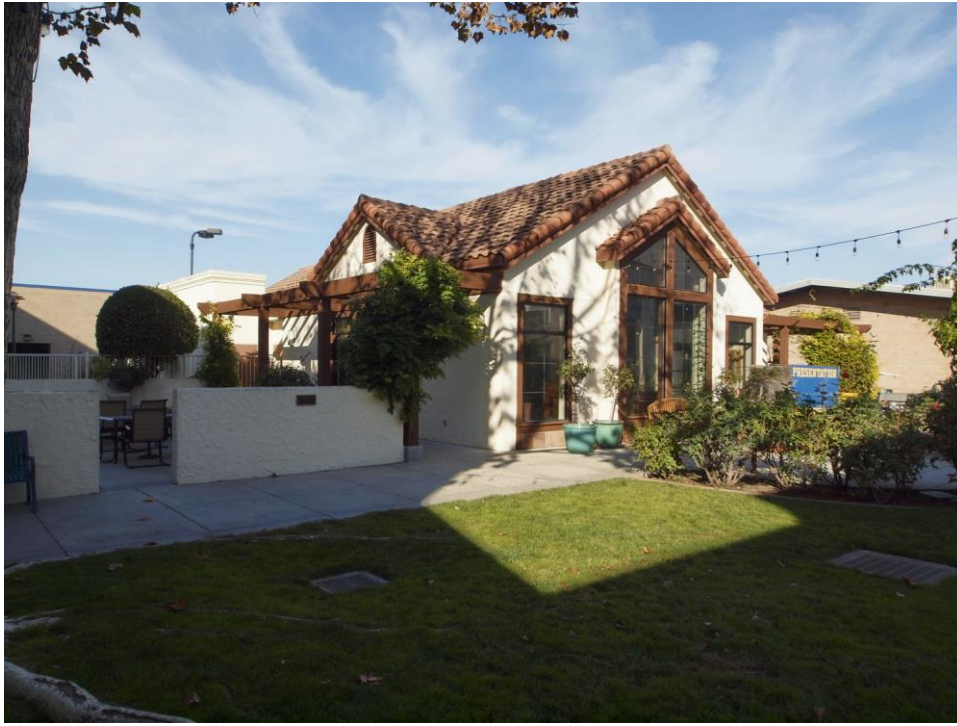
Christian Life Center and Chapel building with courtyard to left, viewed facing northeast.
