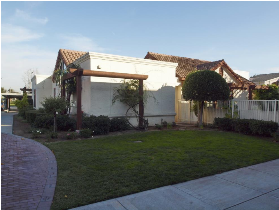
Christian Life Center and Chapel building, viewed facing east.
