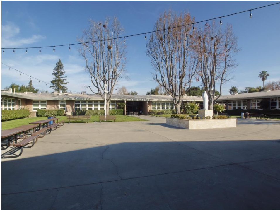
Classroom building from courtyard, viewed facing southeast.
