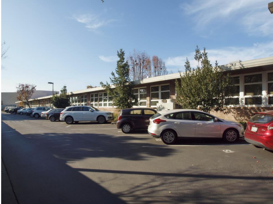
South elevation of main classroom building (south wing) viewed facing northwest.
