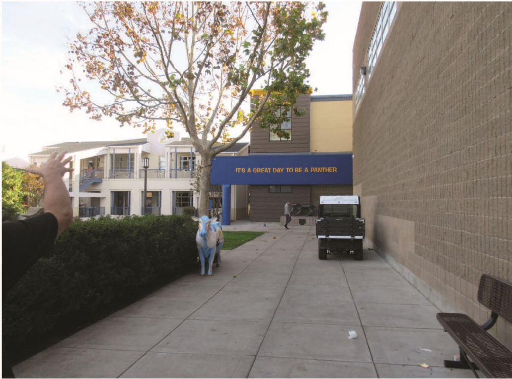
Photo 3: Viewing south across the front of the existing gym building.
