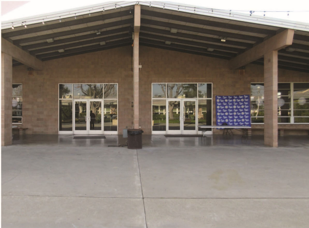
Photo 5: Front side of the existing student center building.
