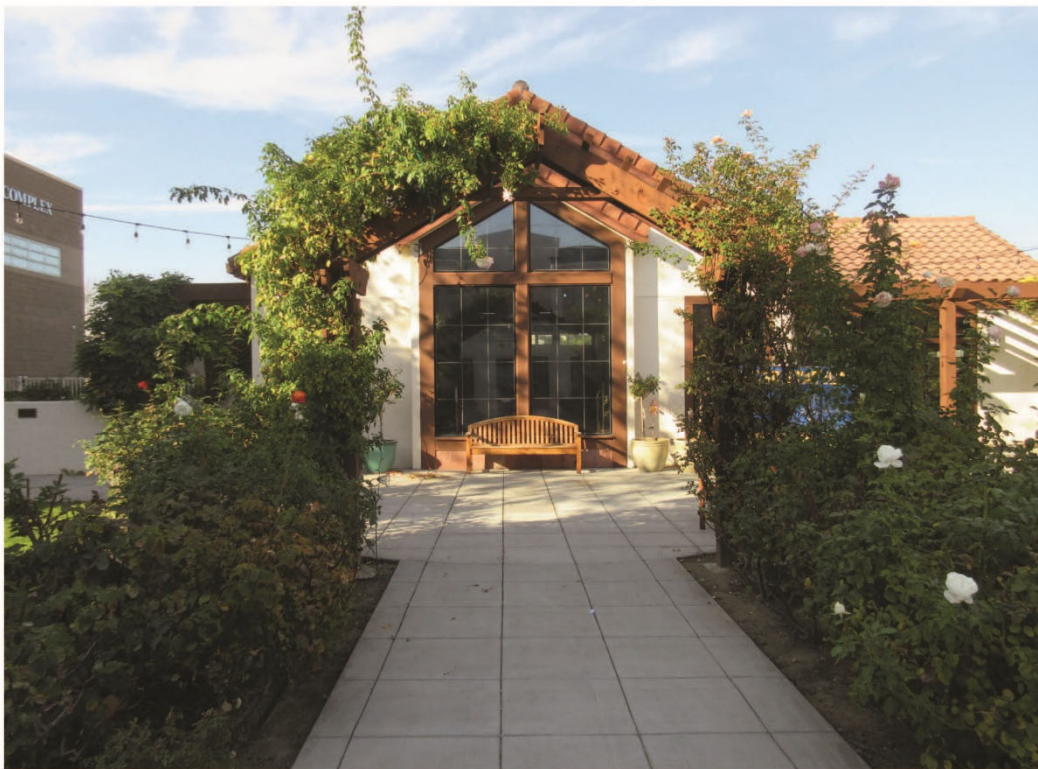
Photo 4: Viewing north toward the existing chapel building.
