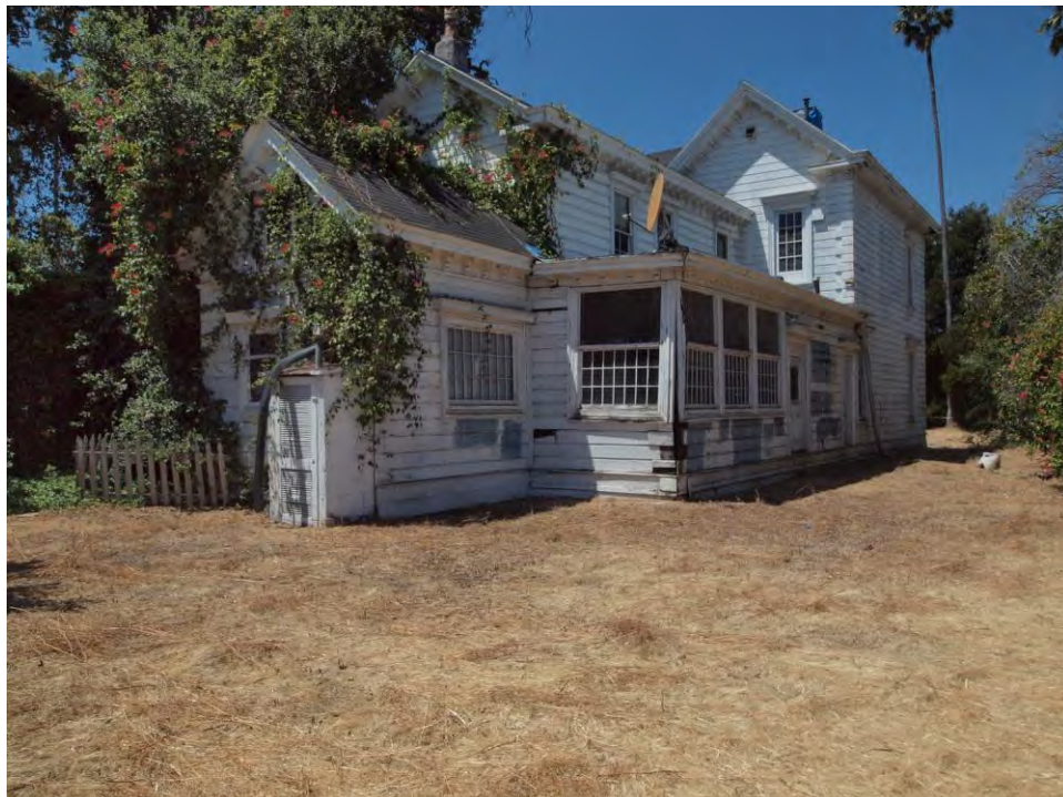
Rear and north side elevations, viewed facing southwest.
