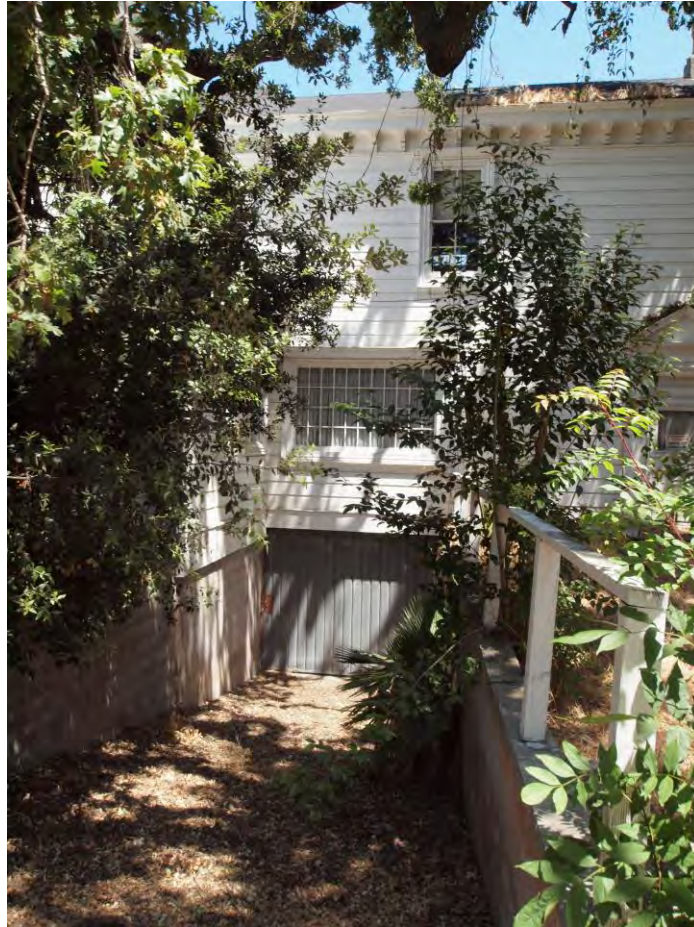
New basement entry at south elevation, viewed facing north.
