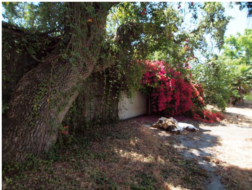
Ancillary building at east property line, viewed facing southeast.
