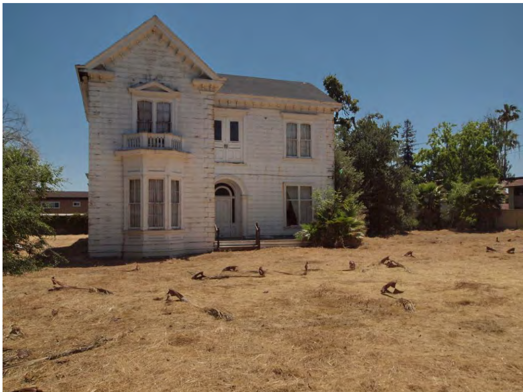
Front elevation, viewed facing east.
