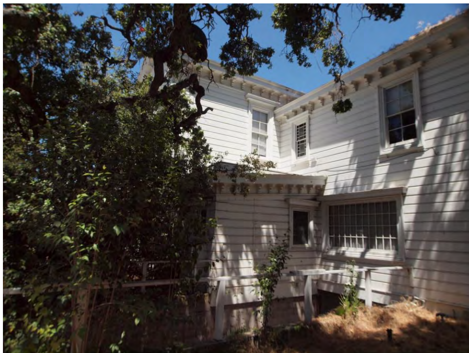
South elevation at rear wing, viewed facing northwest.
