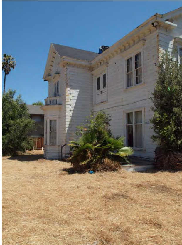
Front elevation, viewed facing northeast.
