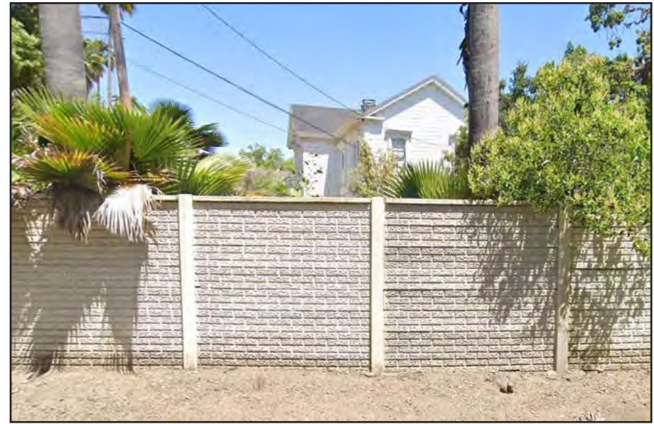
Photo 2. View of the project site from Rancho Way looking north, showing the existing historic building and fencing.
