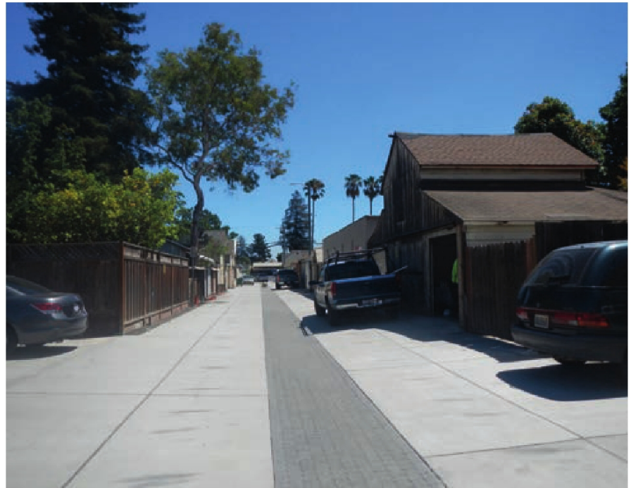
Implementation of GSI measures in the Martha Gardens Green Alleys project significantly improved drainage. The images show conditions before (above) and after (right) project completion. Photo by ESD
