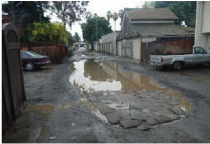
Implementation of GSI measures in the Martha Gardens Green Alleys project significantly improved drainage. The images show conditions before (above) and after (right) project completion. Photo by ESD
