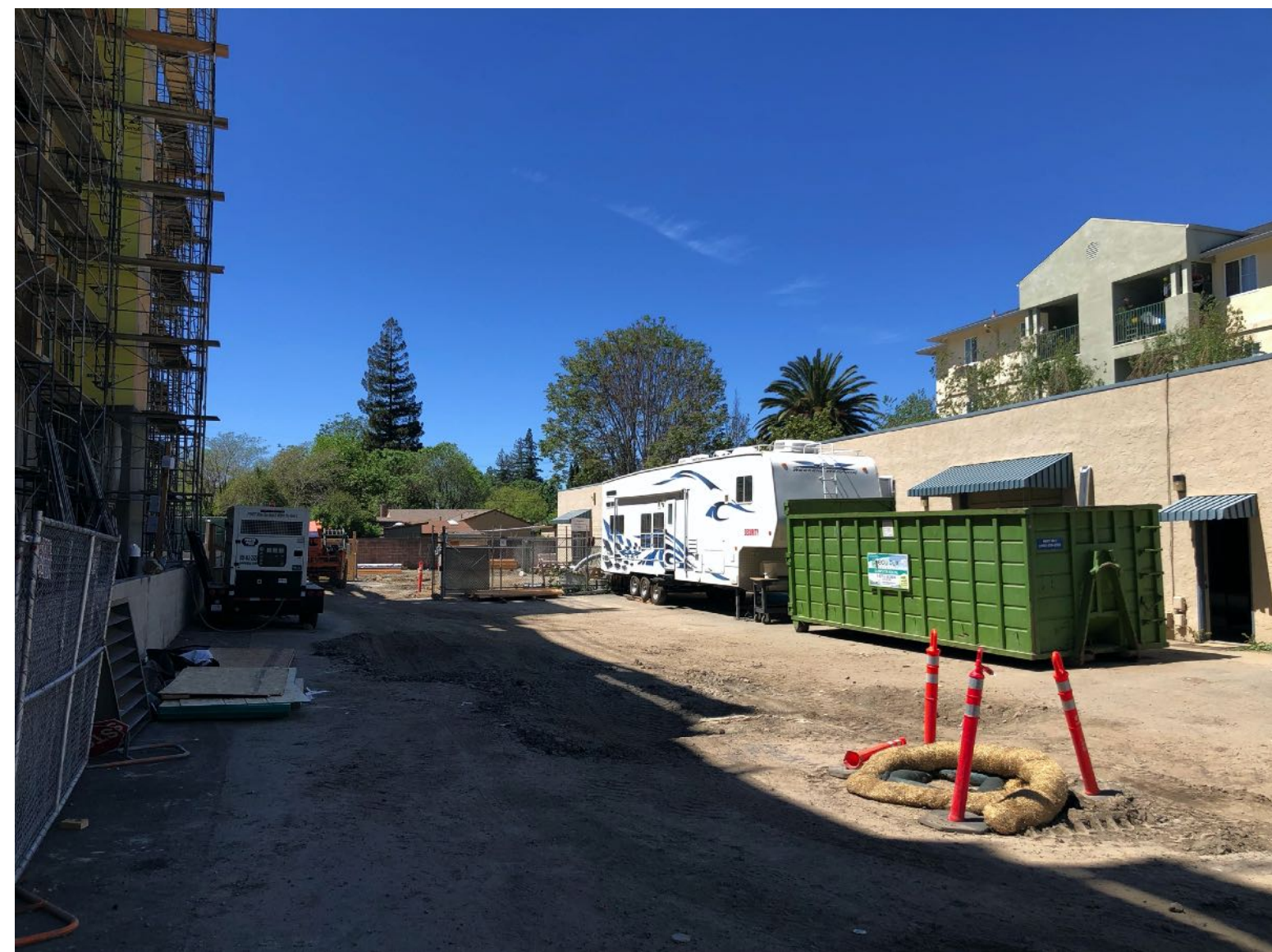
MIDDLE OF SITE TOWARD EAST
