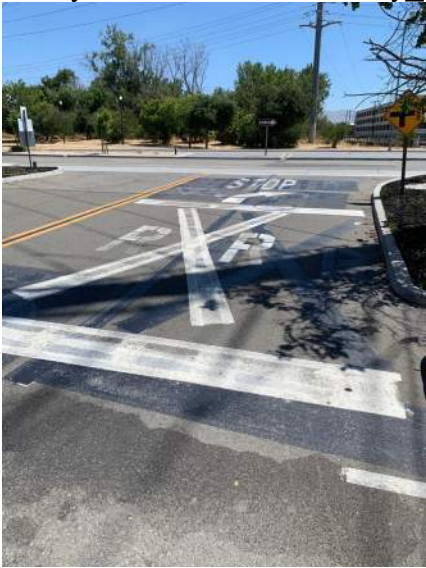
08_Autumn Pkwy Commercial Driveway_facing E.jpg
