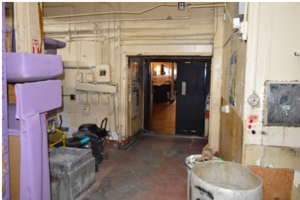
Figure 22. Back-of-house/kitchen area at rear of first story interior, looking southwest.
