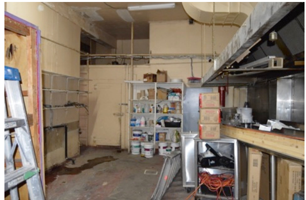
Figure 23. Additional view of back-of-house/kitchen area, looking northwest.
