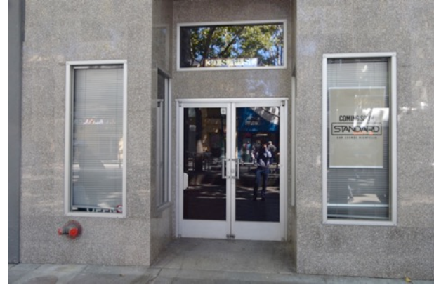
Figure 7. Typical entrance design with double-doors, fixed transom, and adjacent vertical windows, looking east.
