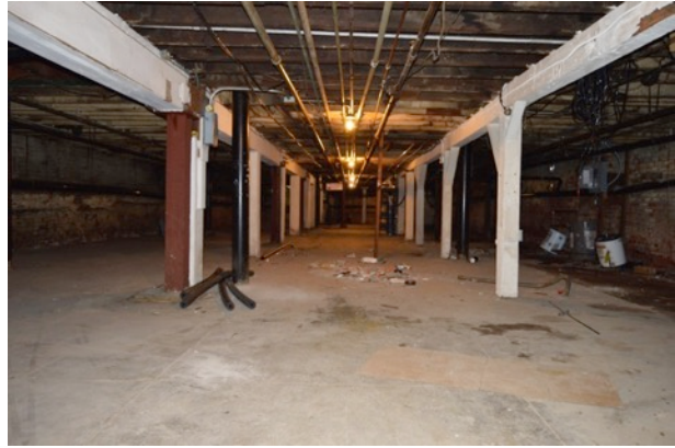
Figure 17. View of basement, looking southwest.
