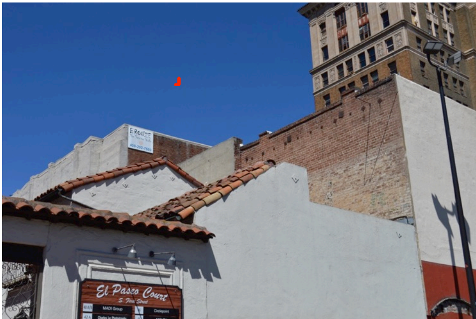
Figure 15. Visible portions of southwest elevation (indicated with red outline), looking northwest.
