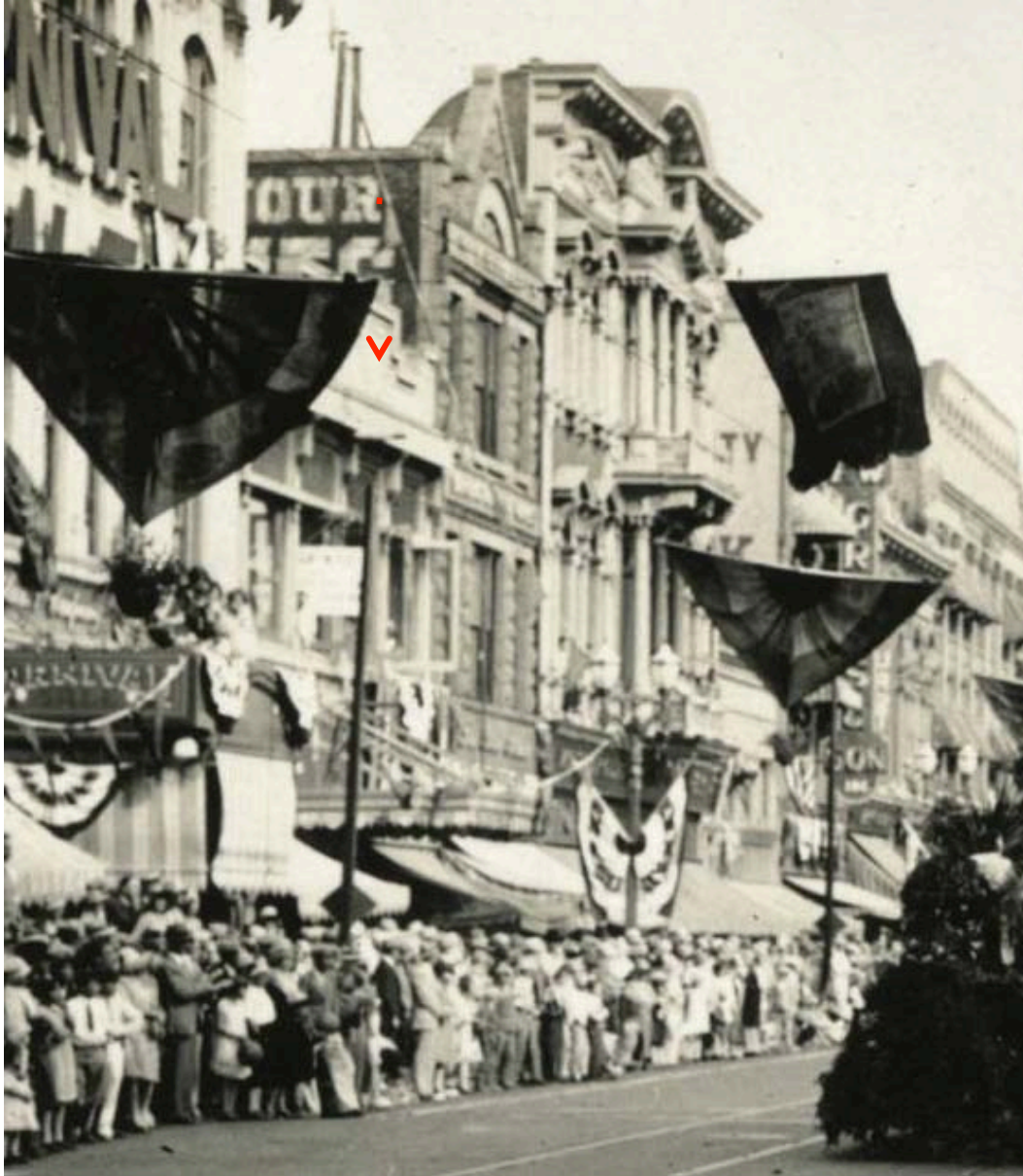
Figure 34. 1928 photograph by Russell E. Pettit of S. 1st Street, capturing subject building (indicated with red arrow) (San Jose Public Library)
