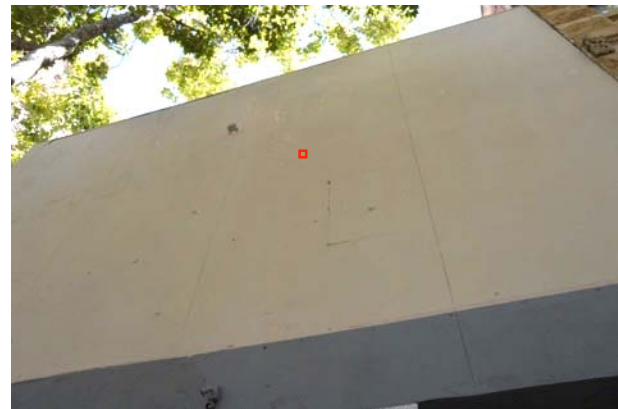
Figure 9. Second story, looking east. In-filled former window opening outlined in red.
