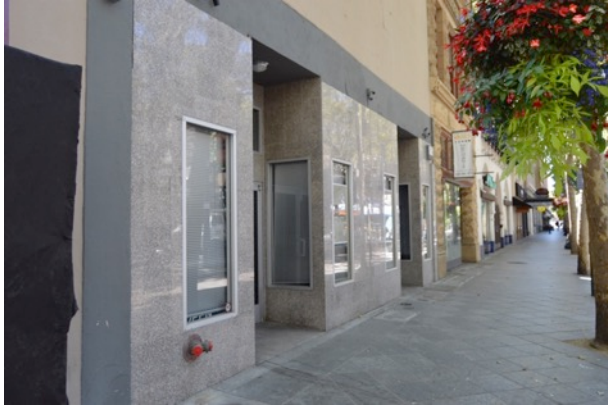
Figure 6. First story, looking west.
