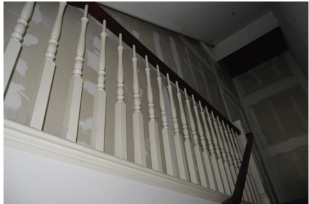
Figure 27. Turned wood balustrade at top of staircase, looking northeast.
