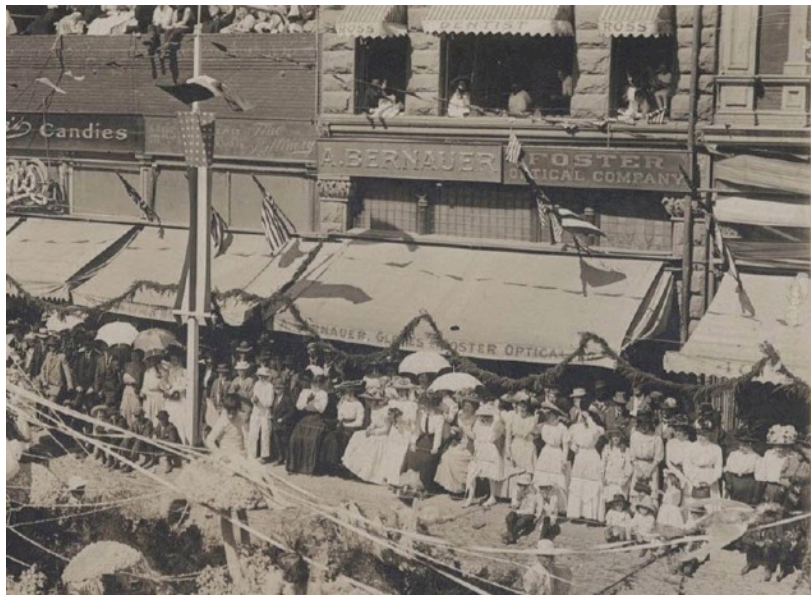
Figure 33. Knox-Goodrich Building (pictured at center), 1910. (History San Jose, Accession 1997-300)
