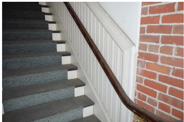
Figure 25. Railing and wood wainscot along staircase at first story, looking southeast.
