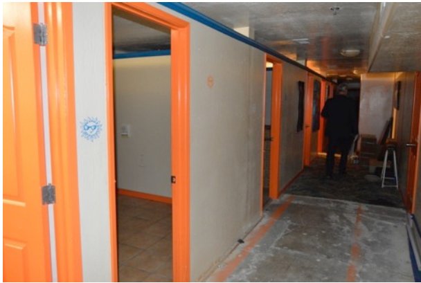
Figure 18. Non-structural partitions within basement, looking east.
