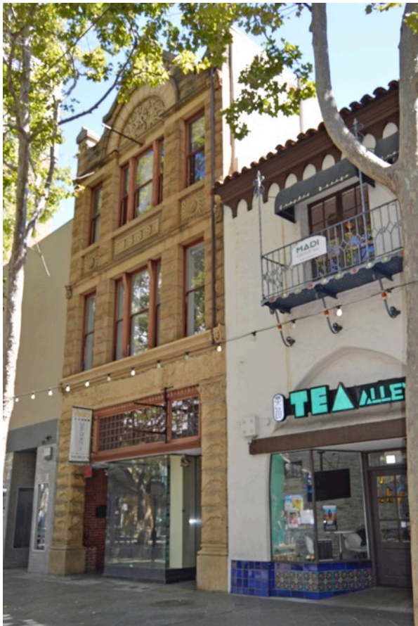
Figure 7. Subject building (left), looking north
