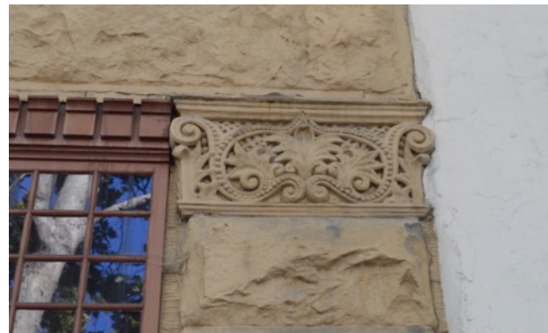
Figure 9. Byzantine capital detail atop first story piers, looking east.
