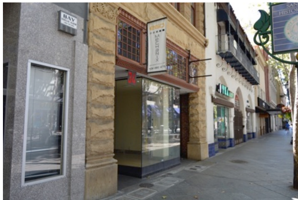
Figure 5. Sidewalk adjacent to front of building along S. 1st Street, looking south.
