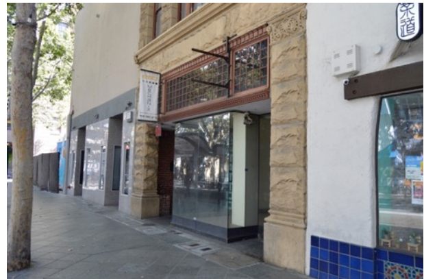
Figure 8. First story storefront and non-historic transom. Piers at this level are clad with simulation sandstone. Looking north.
