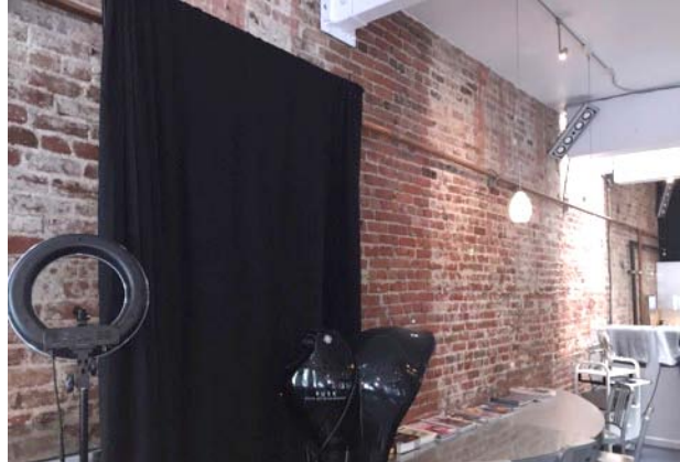
Figure 29. Exposed brick walls at second story, looking west.
