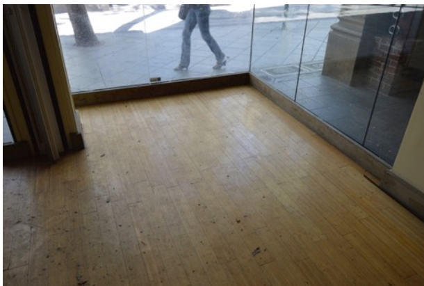
Figure 24. Hardwood floor at front of first story, looking west.
