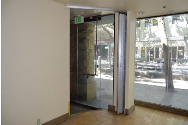
Figure 22. Entrance at south end of building viewed from interior.
