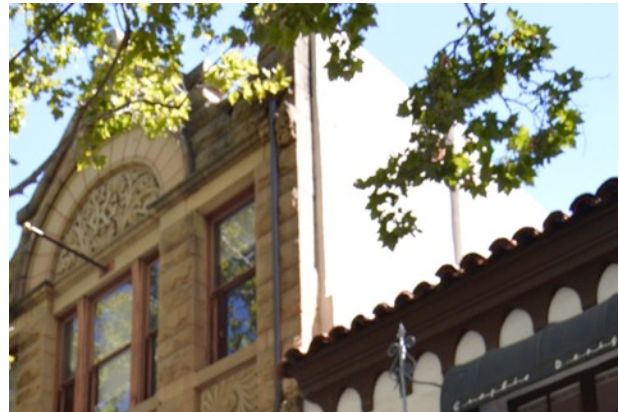
Figure 17. View of front corner of southeast elevation from sidewalk along S. 1st Street, looking southeast.
