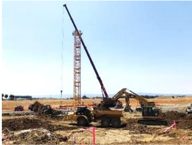
Figure 4 – Start of Headworks 3 excavation and tower crane installation
