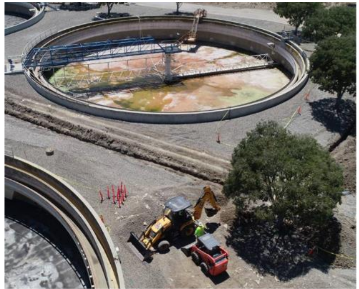
Figure 1 – Trenching between nitrification clarifiers in preparation for an electrical duct bank
