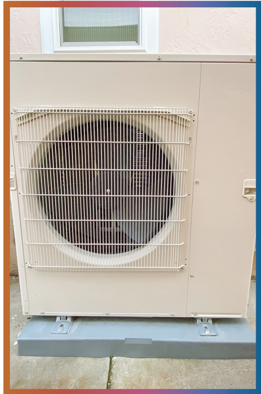
Condenser for a ductless heat pump system installed in a San José home.
