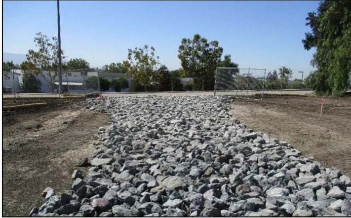
Effective BMPs installed at construction site entrance.
