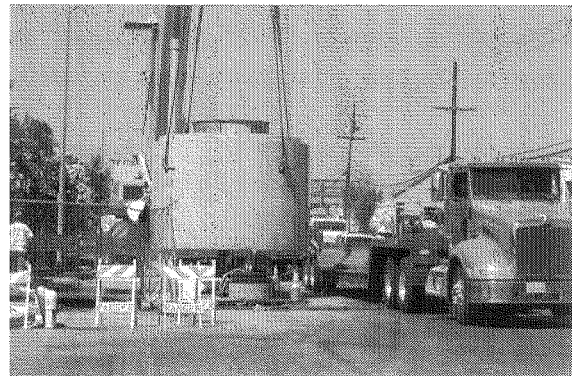
Installation of Large Trash Capture Device on 7 th Street
