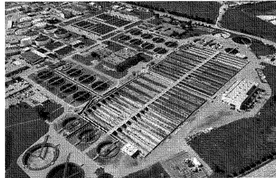
Aerial View of the San José-Santa Clara Regional Wastewater Facility
