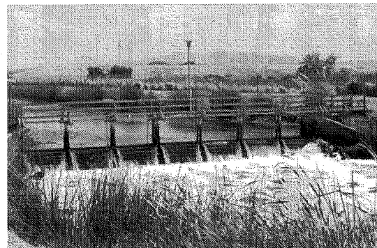
Treated Water Flows to the Bay
