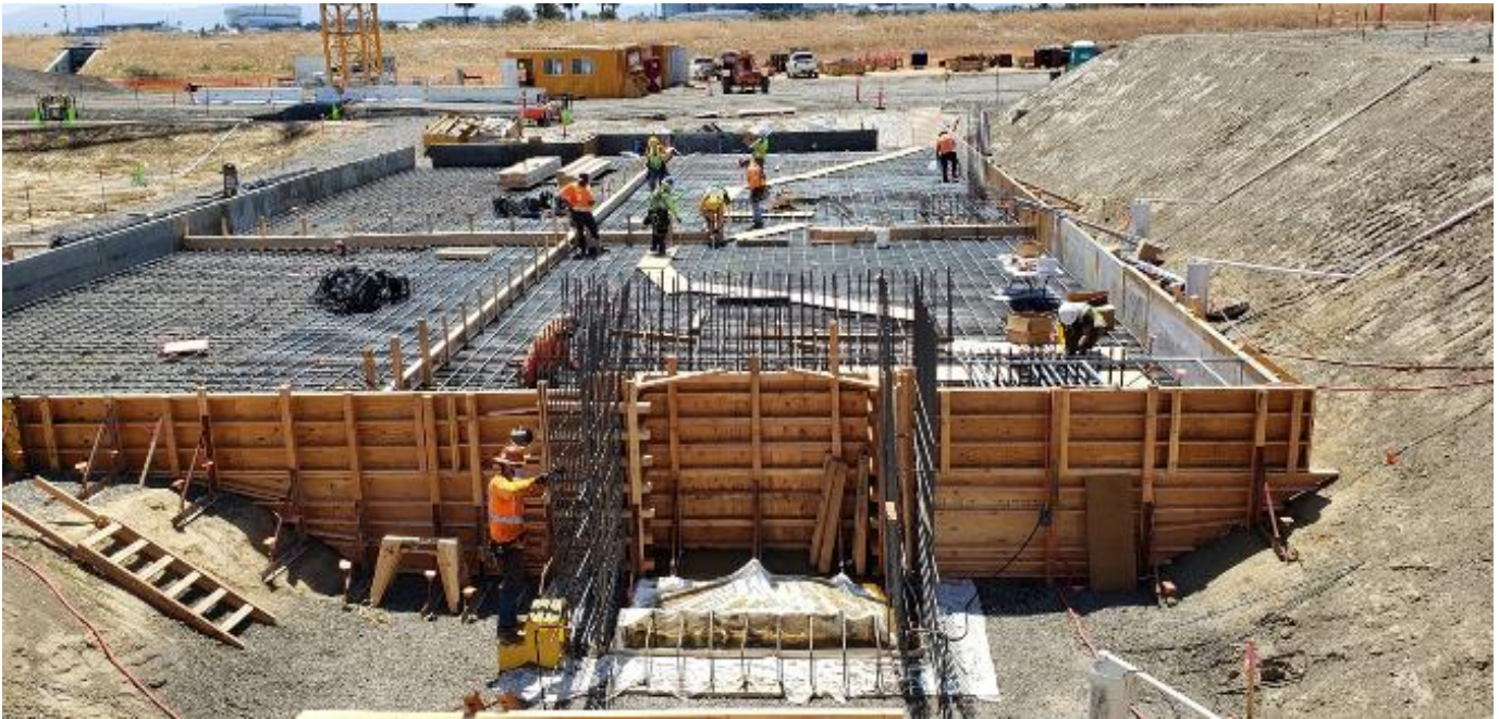
Figure 6 – Installation of rebar for the future Headworks Grit Building
