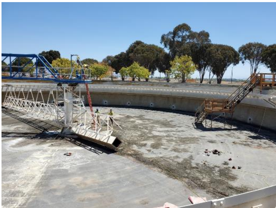
Figure 7 – Nitrification Clarifier B6 demolition
