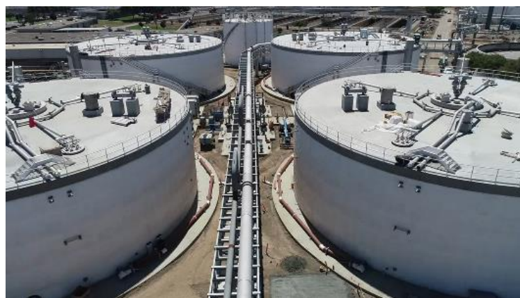
Figure 5 – Digester pipe rack system
