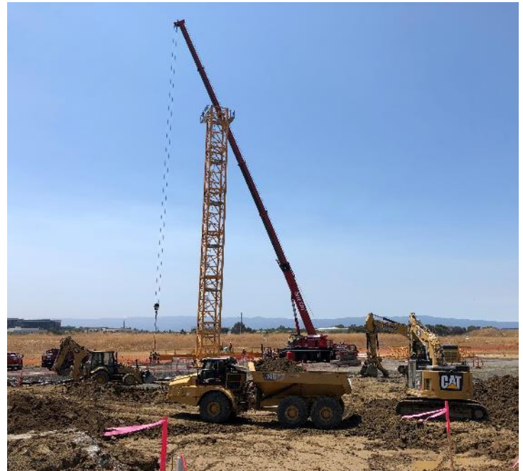
Figure 1 - Headworks mass excavation and erection of tower crane
