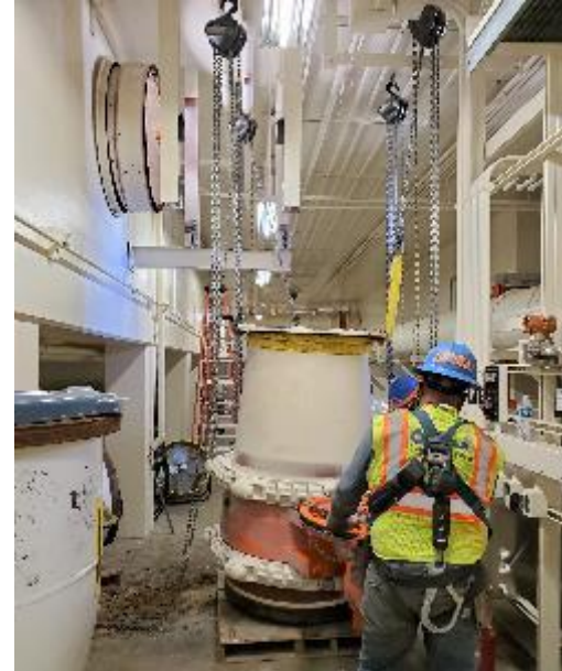
Figure 2 – Nitrification Battery B Tunnel Influent Pipe Demolition
