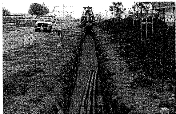
Fire Main Replacement - Phase 2
