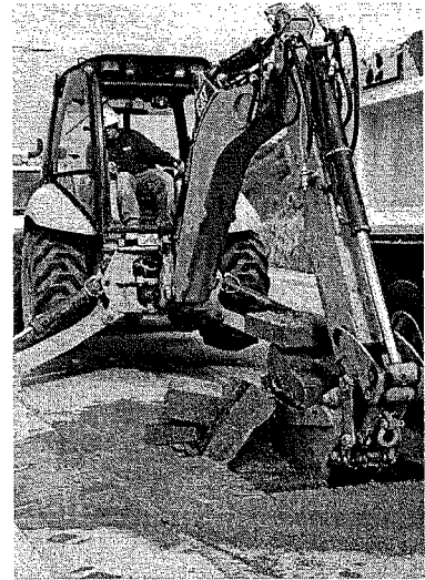
Dove Road Main Extension, completed in 2013-2014
