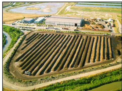
Composting at Newby Island
