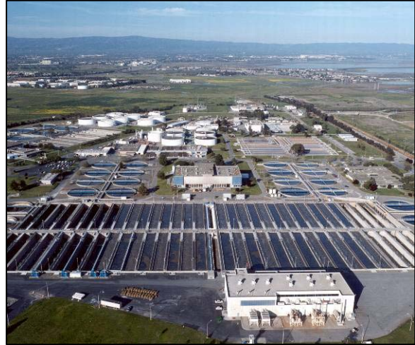
San José/Santa Clara Water Pollution Control Plant
