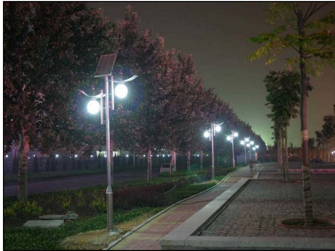
Sample LED pedestrian lighting
