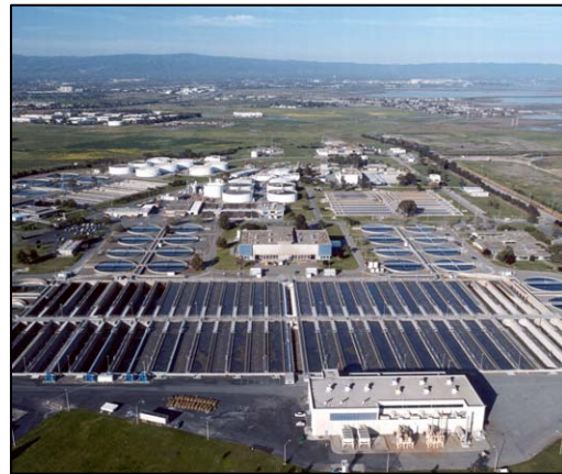
The Water Pollution Control Plant
