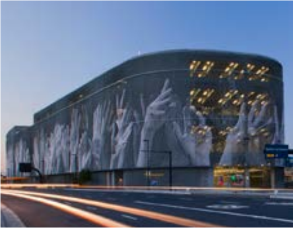
Use visually attractive screen materials San Jose International Airport ©YEI Engineers
