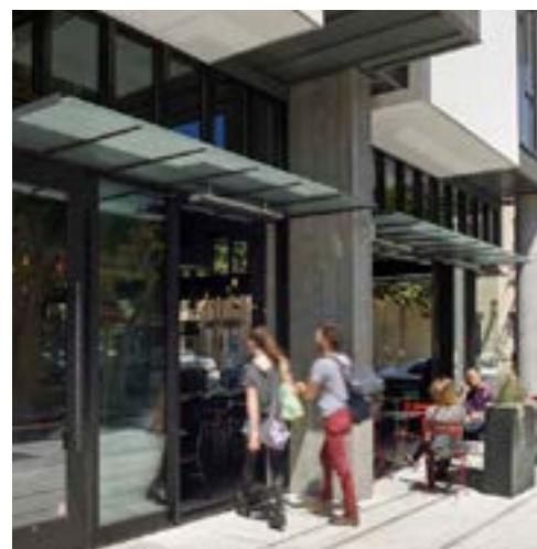
Active Use On Ground Floor © Bruce Damonte
