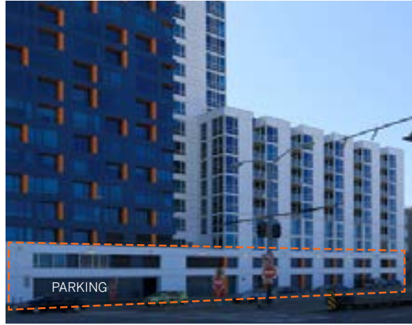
Replicate the adjacent window pattern on a parking garage to mask parking use Source: apartments.com
