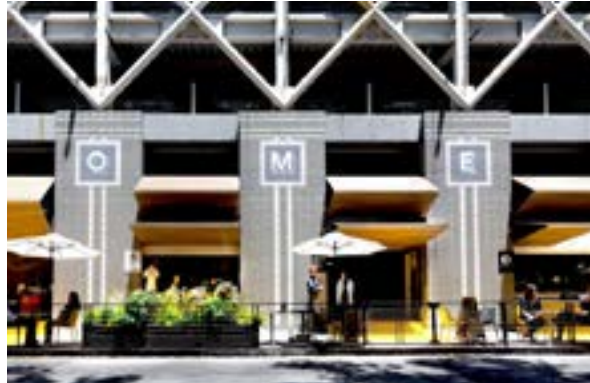
Parking Garage with Ground Floor Retail ©Gensler
