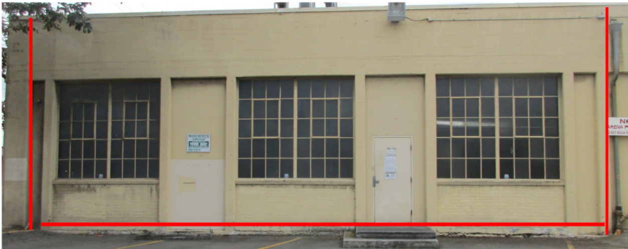
North Wall 50' Section Cut Lines Vertical & Horizontal
