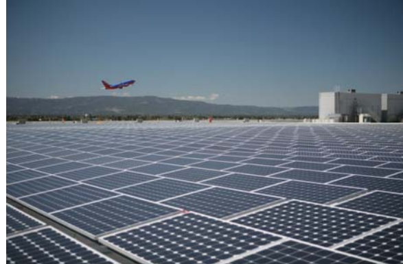
1.12 MW Solar Installation at San José Airport
