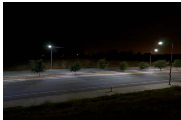
Associated Lighting Representatives - Hadco Evolaire LED Streetlights at Night
