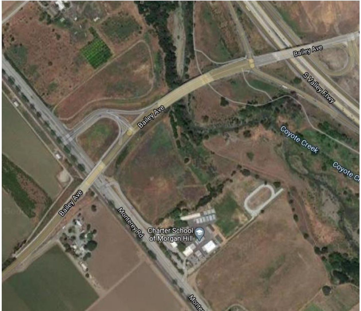
Aerial view of Bailey Ave. cutting through Gundersen property to Hwy 101 Interchange with on and off loop on north side to provide access to Monterey Rd. and frontage road on south side to provide access to Charter School.
