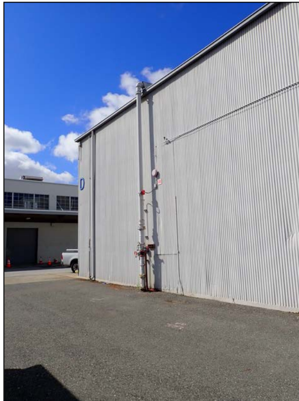
San José Central Service Yard – Building D4. East façade (partial). View to the Southwest. 5/15/20.
