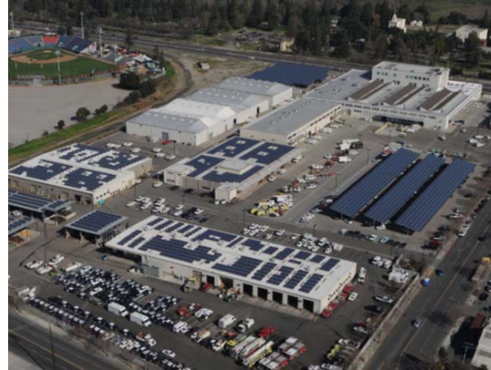
1.24 MW Solar Installation at Central Service Yard
