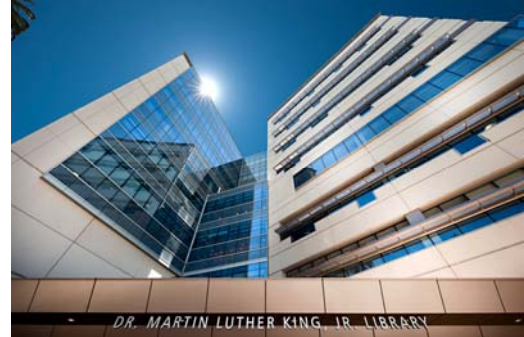
Martin Luther King, Jr. Library - LEED-EB Silver
