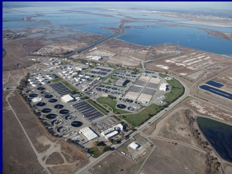
Water Pollution Control Plant
