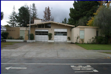
Major Repairs at Fire Stations 4, 14 and 30
