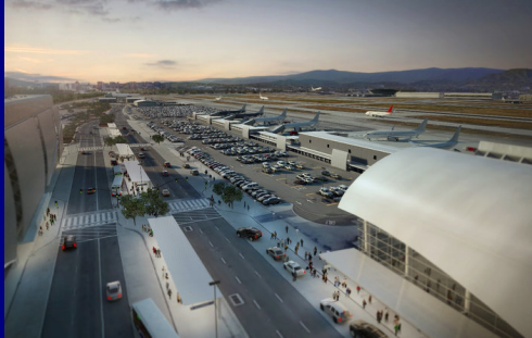
Interim Terminal Facility
