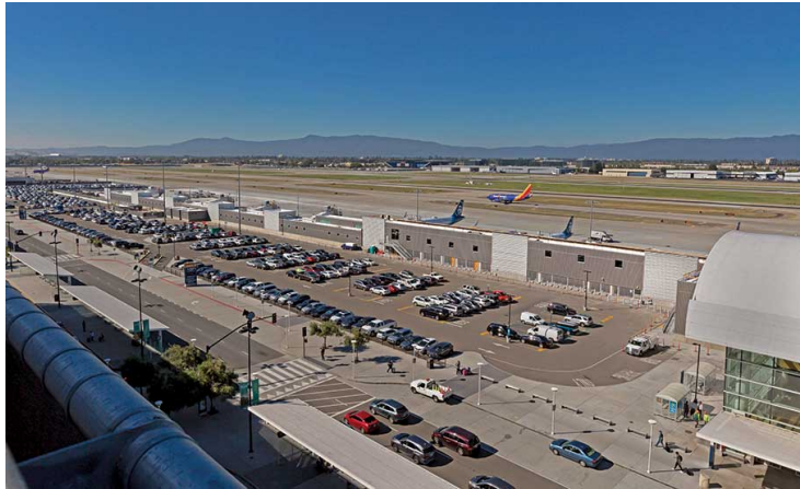
Interim Terminal Facility
